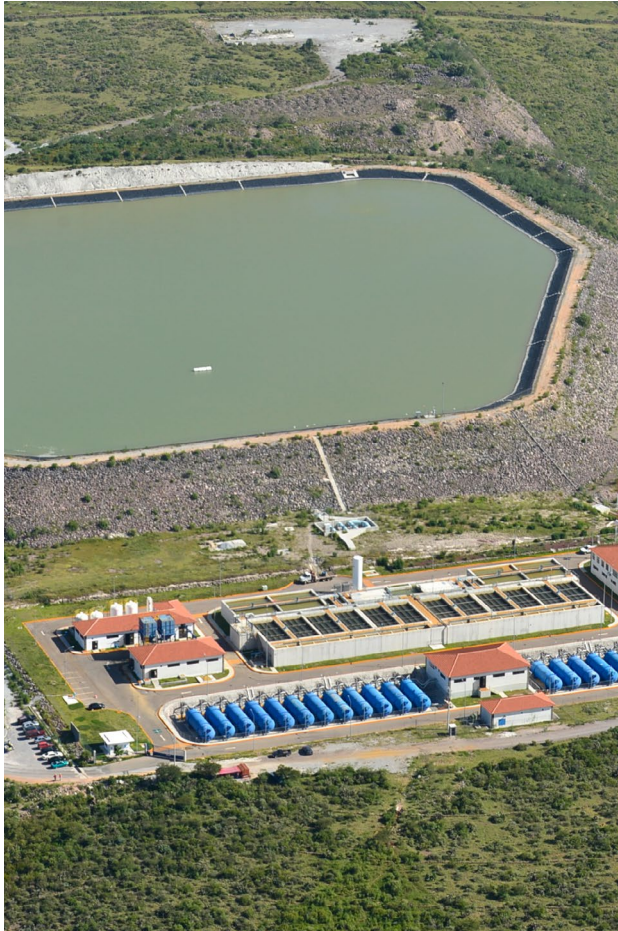
Querétaro aqueduct, Mexico.
