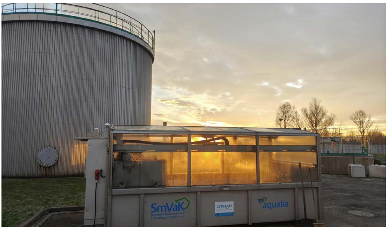
Sludge drying using a solar system.
