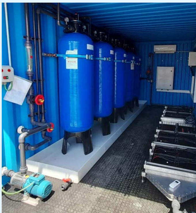
From right to left, skid of continuous and semi-continuous wash filters; and disinfection container with UV, O 3 , and H 2 O 2 .
