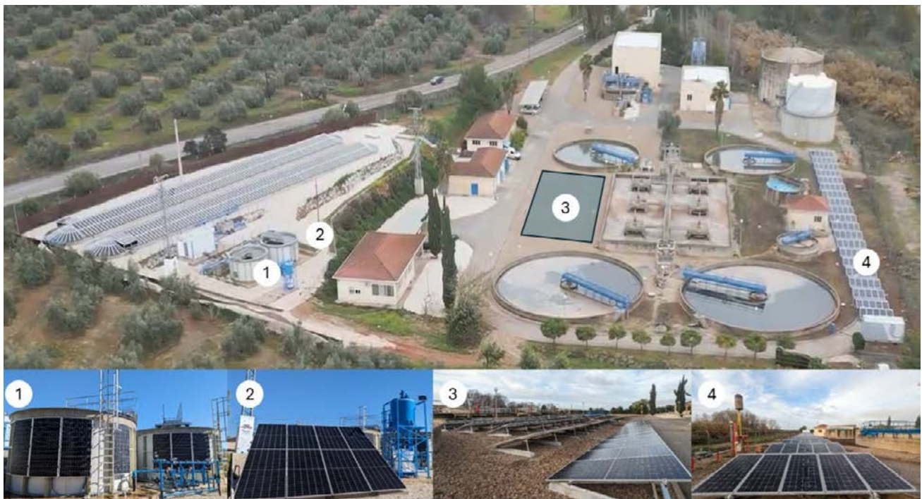
Aerial view of the Linares (Jaén) WWTP and distribution of the incorporated innovative panels:
