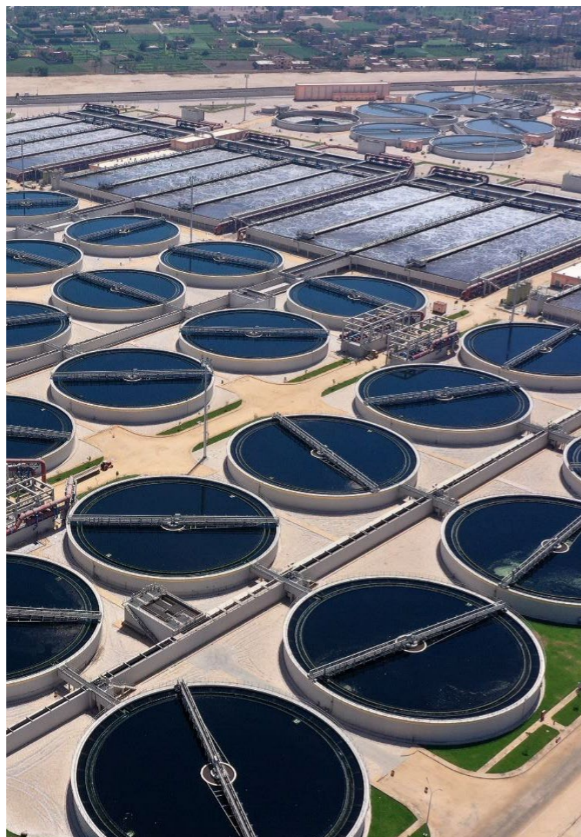
● Abu Rawash WWTP in Cairo (Egypt).
