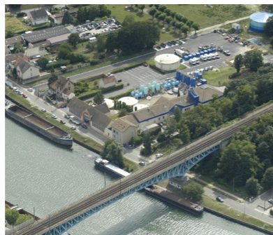
● SEFO facilities in Andresy, France.
