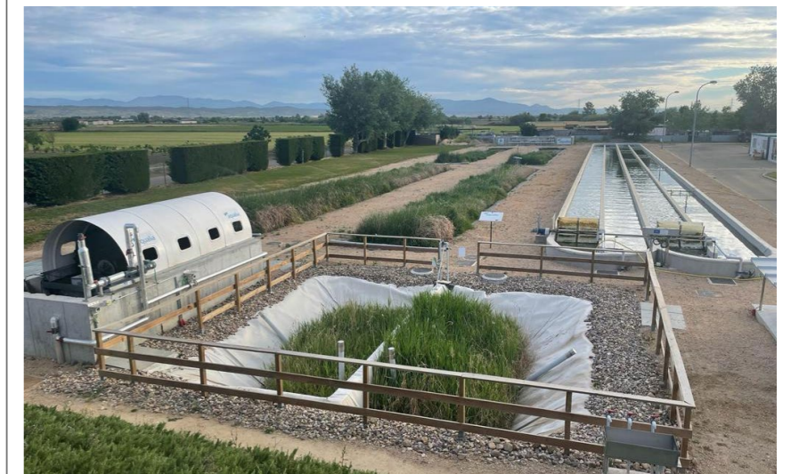
● INTEXT project at the Talavera de la Reina WWTP, Toledo, Spain.
