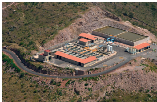
The Water Treatment Plant of El Realito (Mexico)
