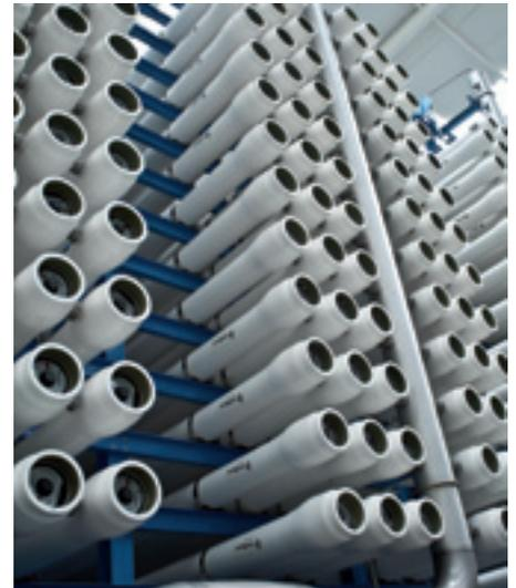
Membrane frame at Cap Djinet desalination plant.
