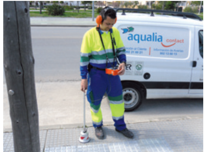
FCC Aqualia personnel performing leak-detection tasks.
