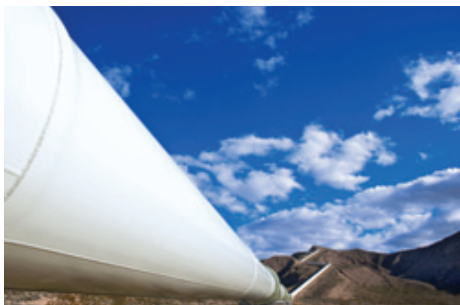
Realito Aqueduct, Mexico.
