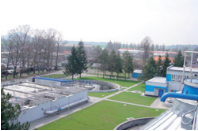
WWTP of N.Jiin (SmVaK).
