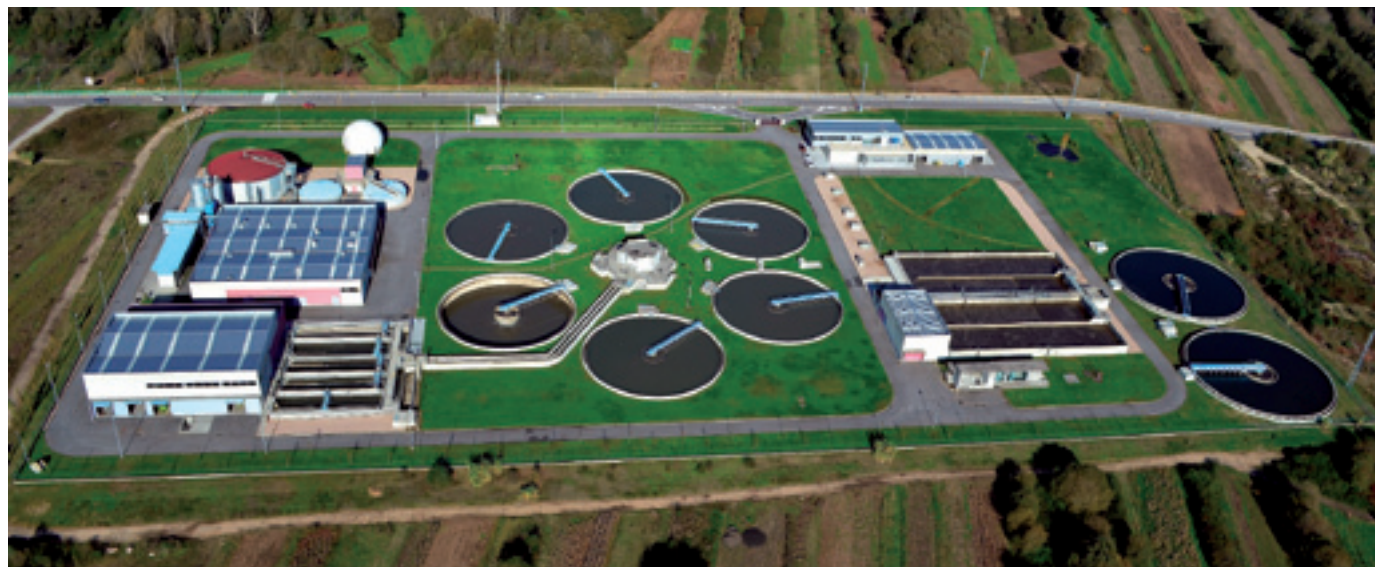
Aerial view of the WWTP Guillarei where the ELAN® process that reduces the energy cost of purification is carried out.
