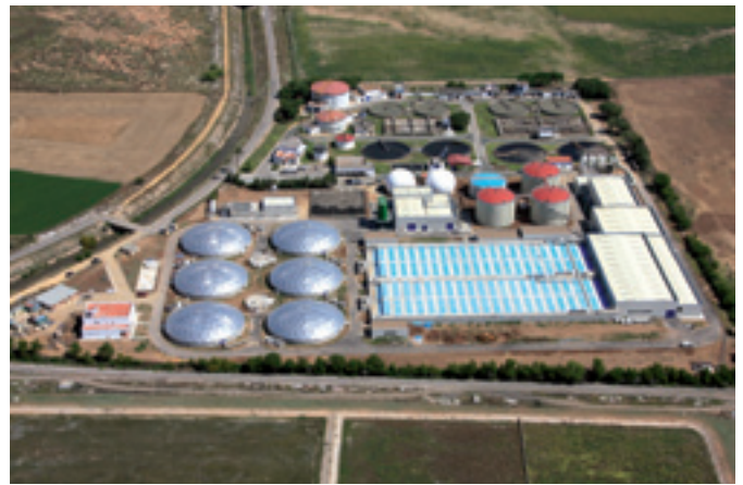
Aerial view of the WWTP La Ranilla.
