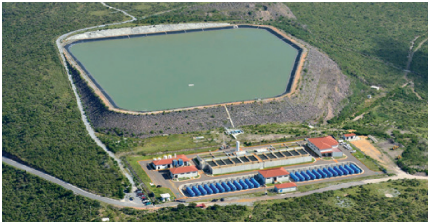
Aqueduct and Aqueduct II treatment plant, Mexico
