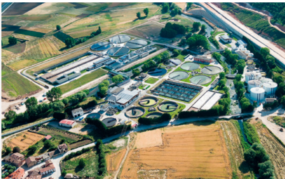
Aerial view of the Burgos WWTP.
