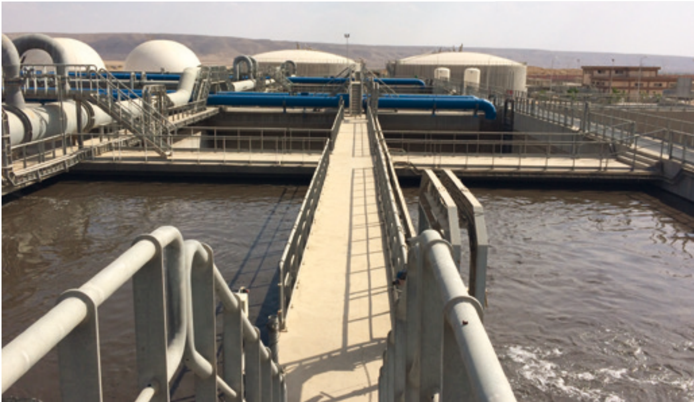
New Cairo Wastewater Treatment Plant.
