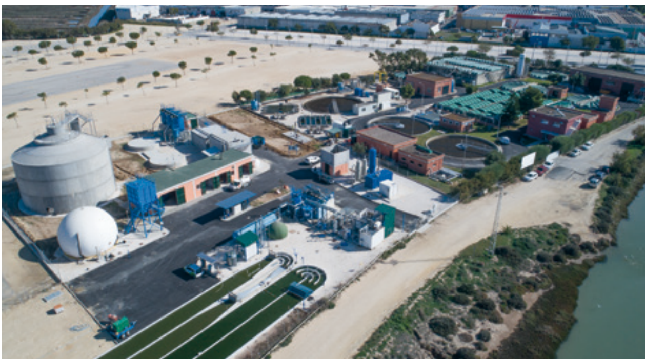
Aerial view of Chiclana WWTP.
