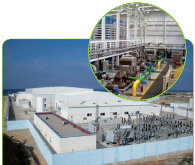
Cap Djinet (Algeria) - 100,000 m 3 /d, exterior and interior.
