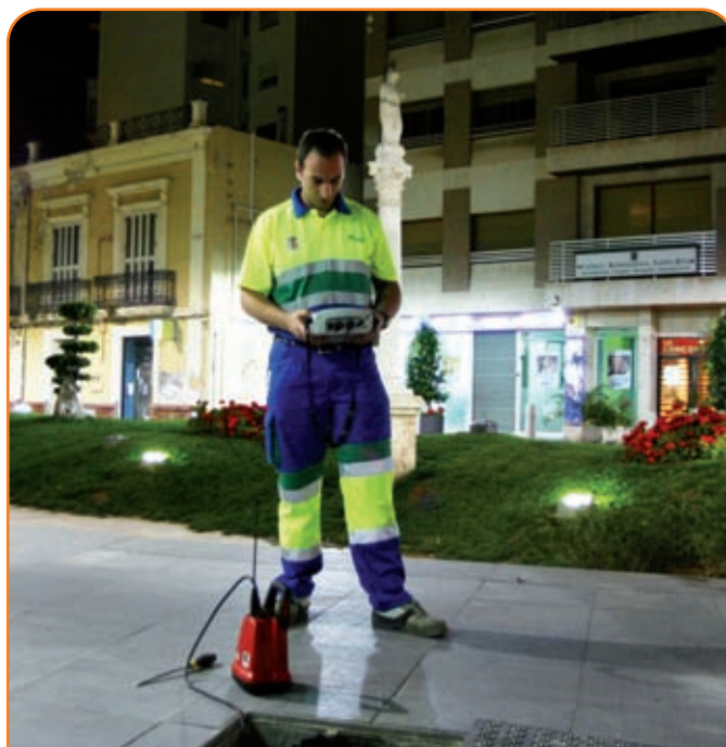
aqualia operative locating leakages.
