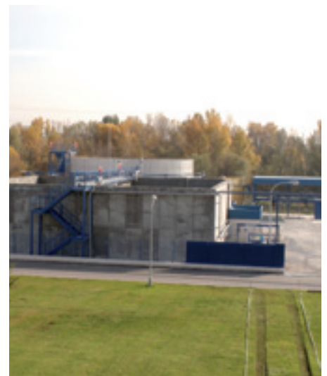
Wyeth treatment plant.
