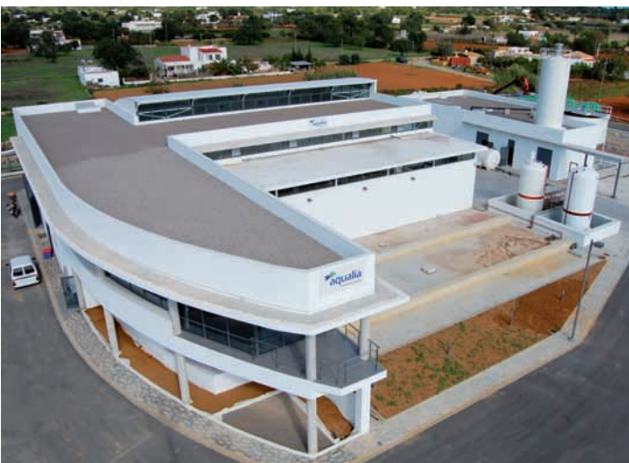
Desalination plant in Santa Eulalia (Ibiza).
